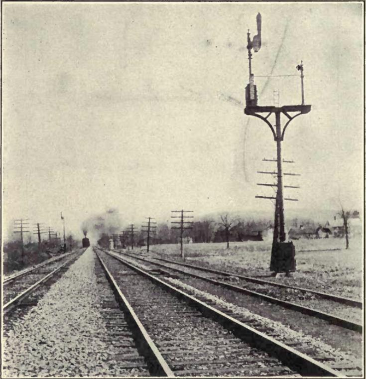
FIG. 14.—Bracket signal and doll post.
