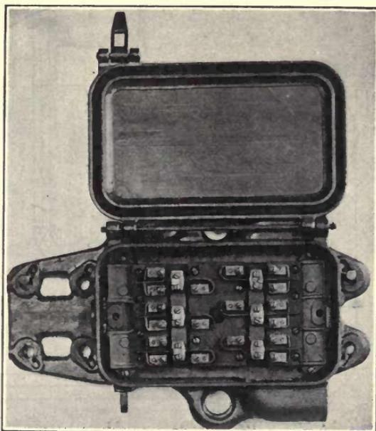
FIG. 105.—Pole-changing indication circuit controller.
