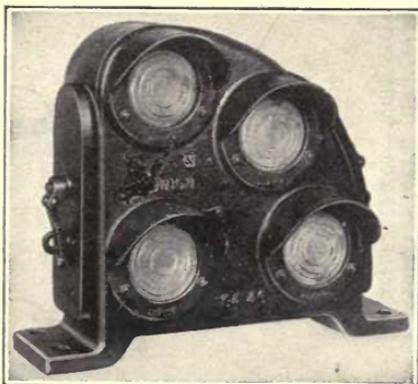
FIG. 318.—Position-light dwarf signal.
