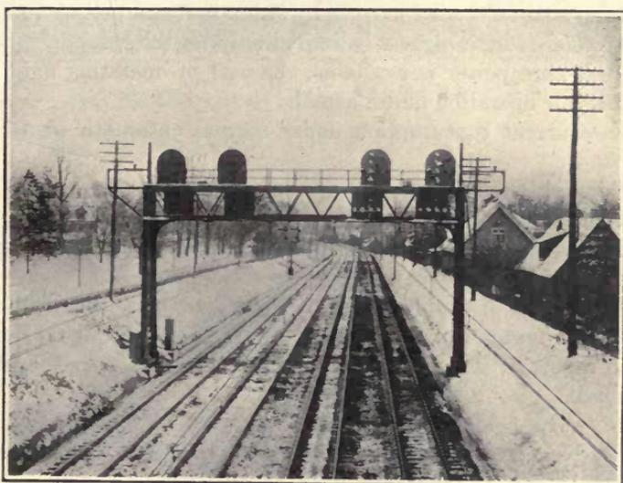
FIG. 6.—Position-light signal.
